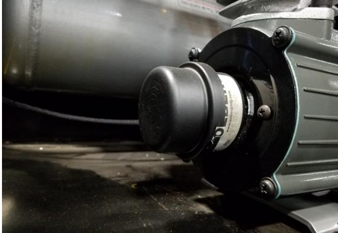
Figure 52: Air filter on compressor.
