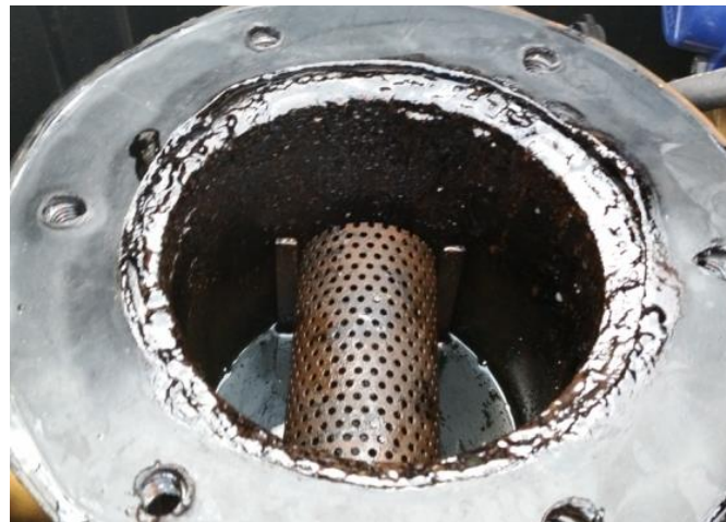
Figure 50: Strainer screen in the pumping station
