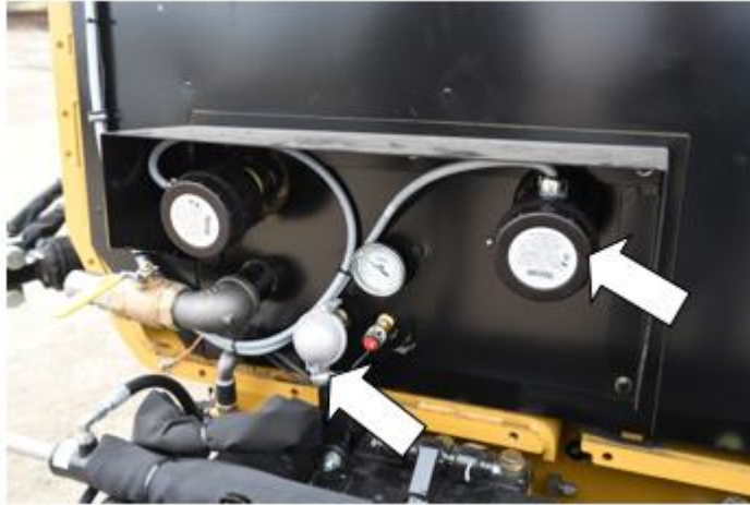
Figure 20: Tank heating elements and thermostat temperature sensor
