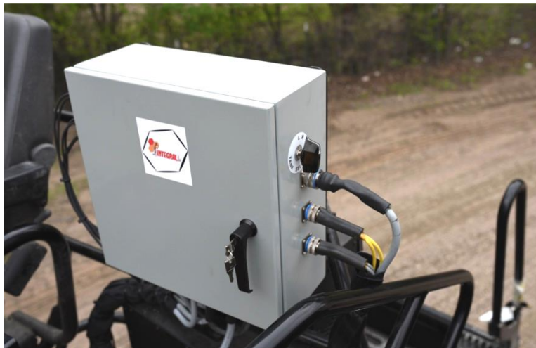
Figure 28: Main control box
