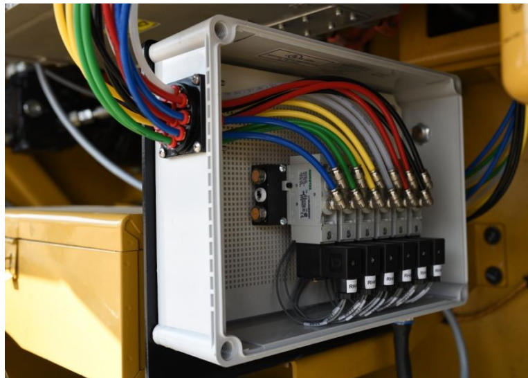
Figure 20: Solenoid valve manifold in its enclosure
