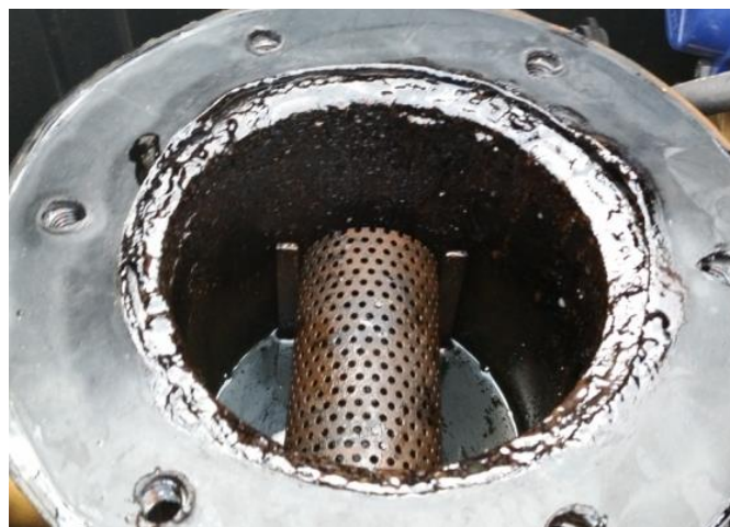
Figure 43: Strainer screen in the pumping station
